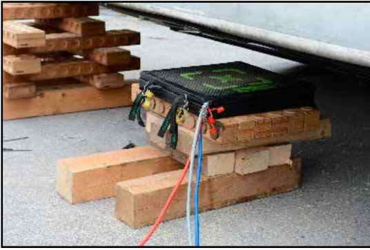
Fig. 5.2: Positioning a SAVA lifting bag on site
